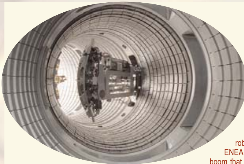
Installation of a sector of the toroidal limiter inside the FTU vacuum chamber
