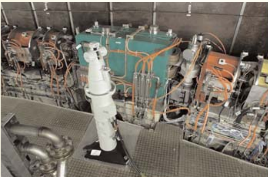
Alignment of the magnets at the Elettra synchrotron of Trieste
